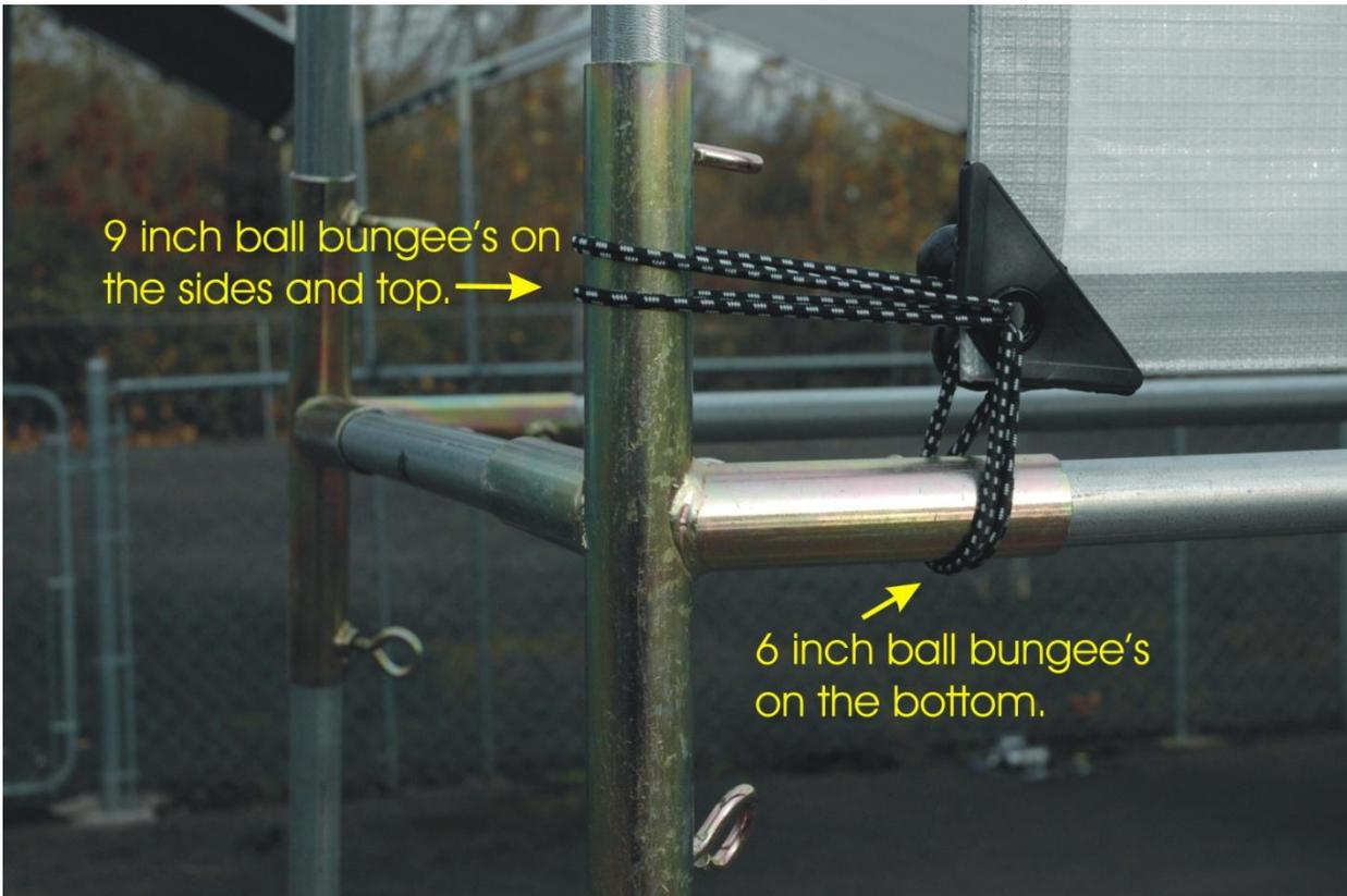
Figure 15 - Proper way to attach bungees to corner of tarp
