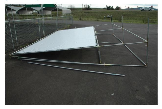
Figure 7 - Screen attached and ready to set upright
